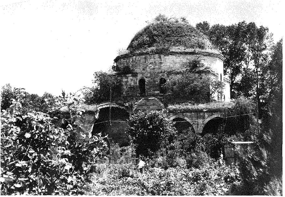
1. Serres, Mehmed Bey Mosque, (1492). The open portico has collapsed in recent years.
